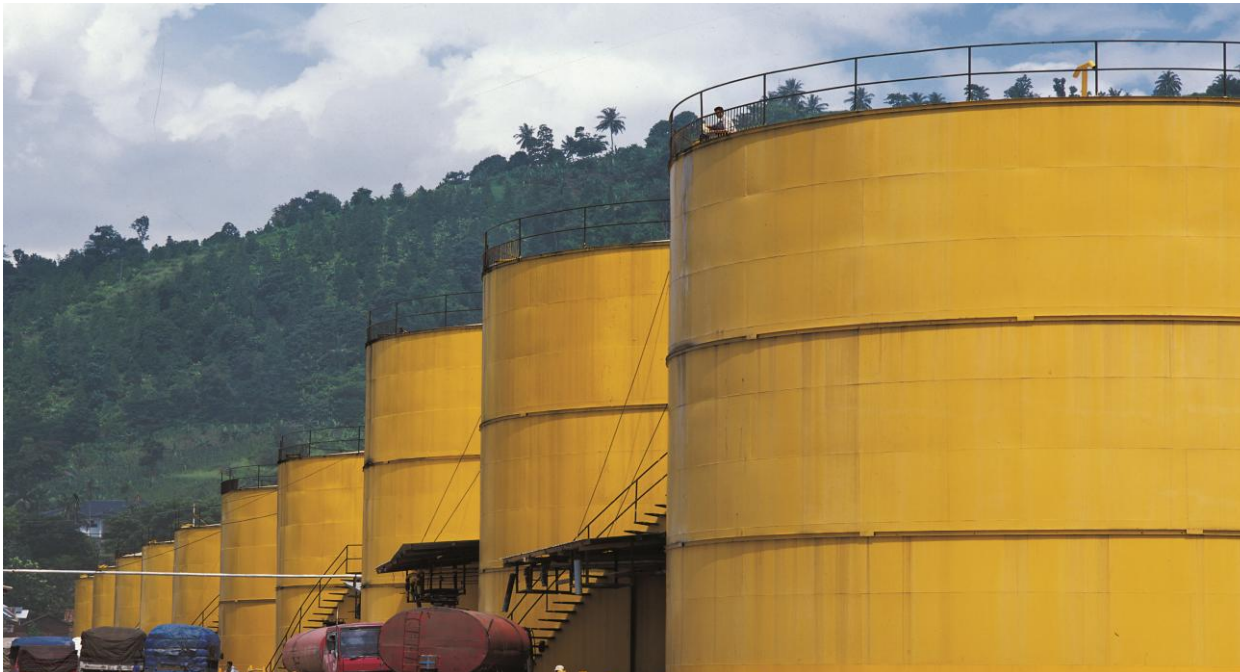
Image: Silos at TBLA's plant, Lampung
