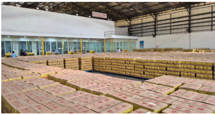
Figure 74. TBLA Cooking Oil Storage Facilities
